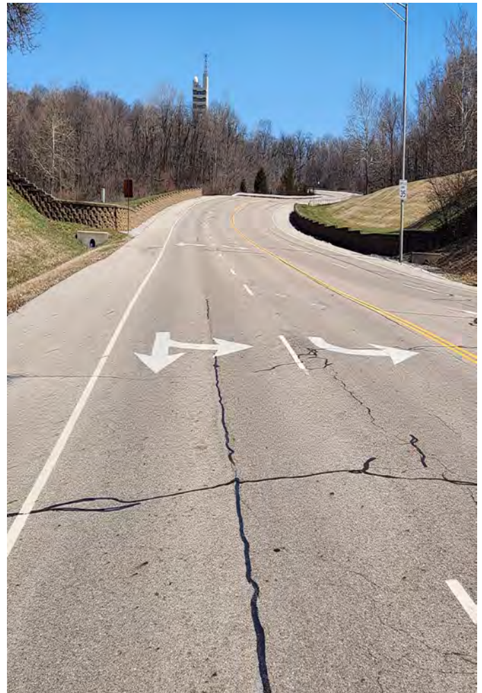
Loop Road Looking East
